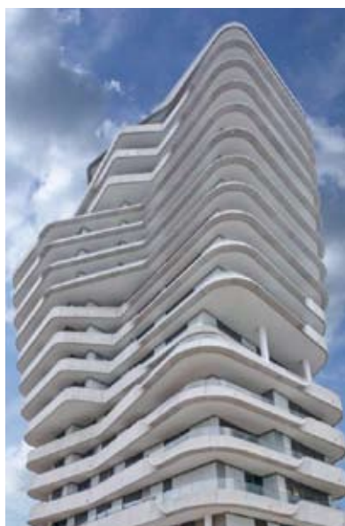
Referenzobjekt: Marco-Polo-Tower, HafenCity Hamburg
